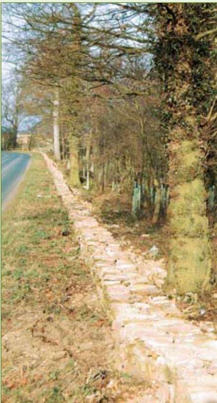
Restoration of a section of Wiganthorpe Park wall. Capstones will be added soon to protect the wall from weather erosion
