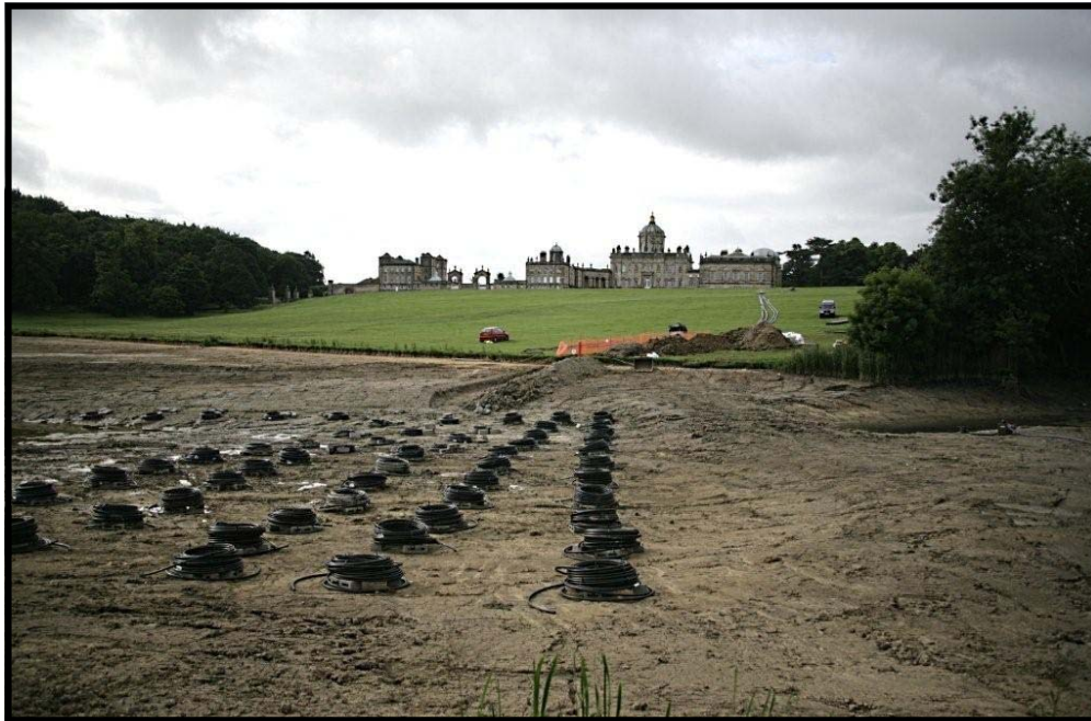
Ground source heat being installed at Castle Howard
