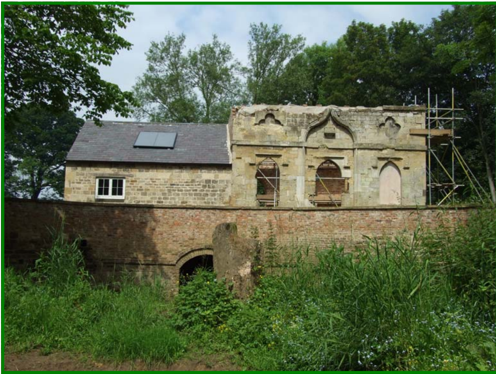
Solar panel on the roof of the granary at Howsham
