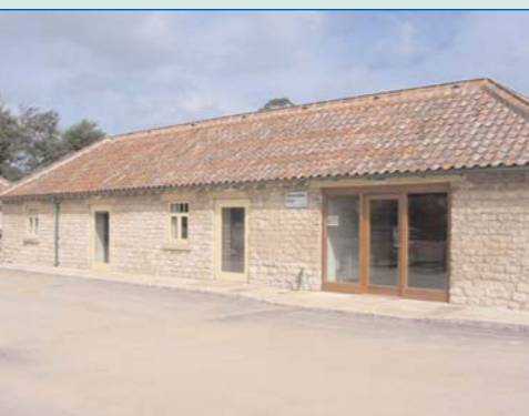
New AONB Office, Hovingham.
